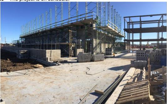
**PERFORMING ARTS CENTER** (PAC) – Block walls are being erected at the PAC stage, the stage fly loft and back of stage. The three story classroom building is beyond and to the right.
