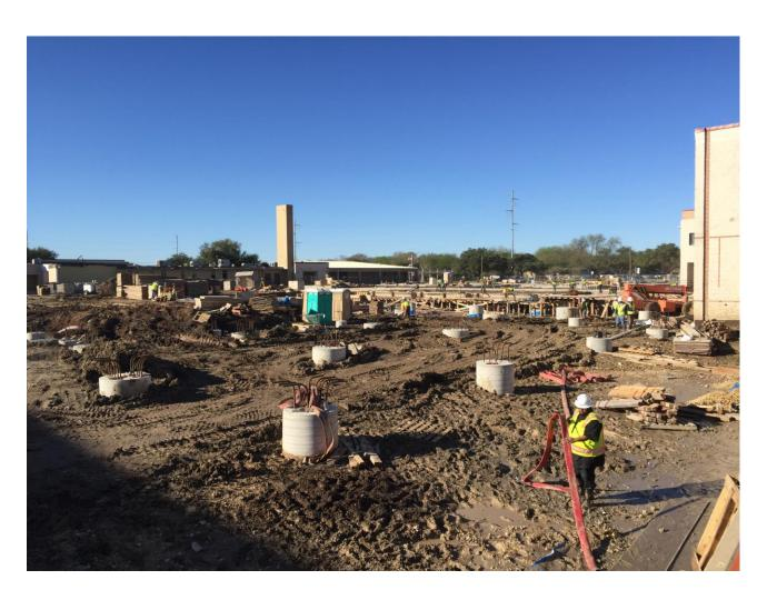
CAREER TECHNOLOGY AND ART ROOMS - The concrete foundation has been poured at the Career and Technology Classrooms. Inclement weather has impacted the concrete pour scheduled for this week at the Art Rooms. The foundation formwork will continue this week.
