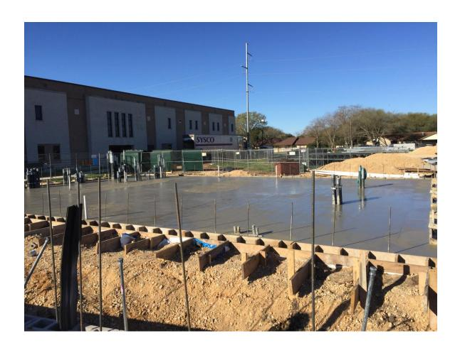
**CHILLER BUILDING** – The concrete foundation for the chiller building was poured this week. This building which is located immediately north of the Freshman Center will house the mechanical equipment for the school.
