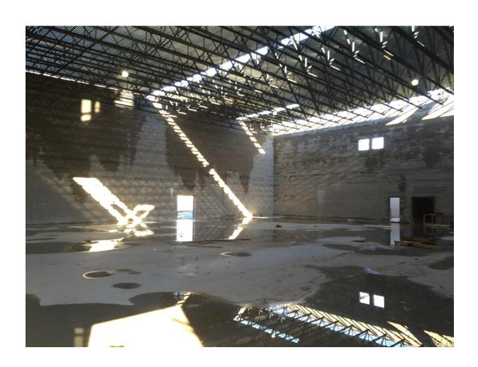
**GYMNASIUM** – Steel roof decking installation is in progress at the Auxiliary Gym.
